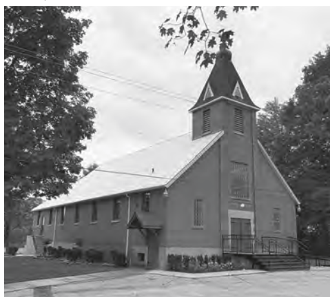
Exterior of the newly renovated Courtland church
